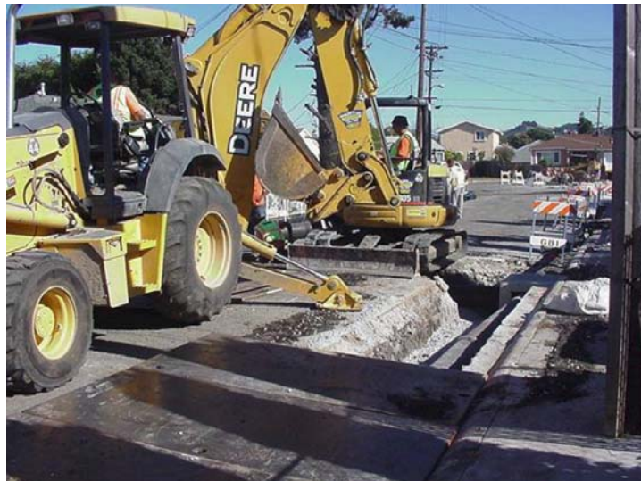
New storm drain
